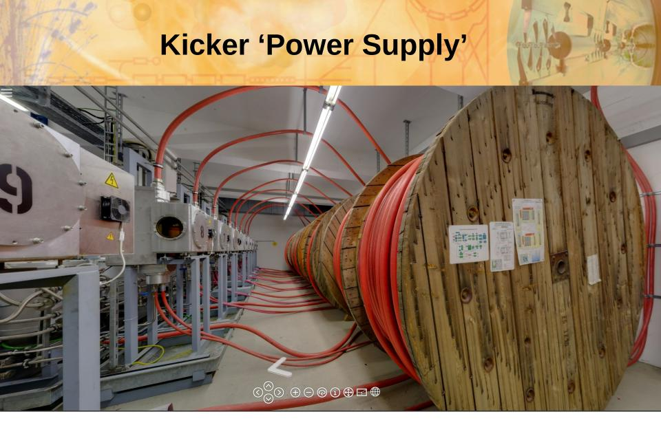
1. pre-fire ( $\sim$ 1  $\mu$ s): discharge capacitors  $\rightarrow$  'transformer+electron tubes'  $\rightarrow$  high voltage  $\rightarrow$  charge cables 2. fire:  $\sim$  1 $\mu$ s later, discharge cables via electron tubes
